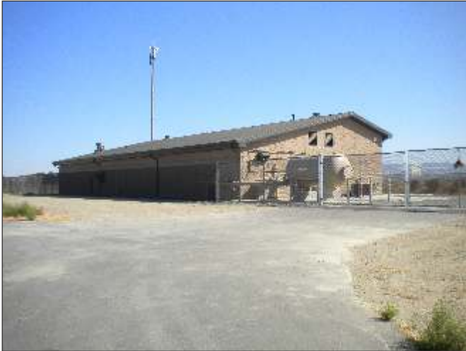
Photograph 3: Pump station adjacent to Lake H.
