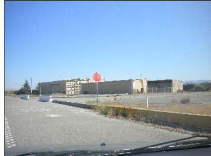
Photograph 4: Former storage sheds before Busch Gate.
