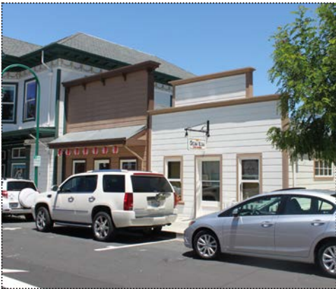
Pinkley Tin Shop was moved to the rear of 600 Main Street. The rear portion was demolished and reconstructed in 2004 (ARG, June 2012).
