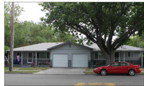
Post-war residence at 104 Abbie Street (ARG, June 2012).
