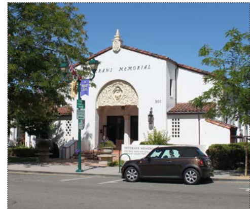
The Veteran's Memorial Building at 301 Main Street was built in 1933 (ARG, June 2012).
