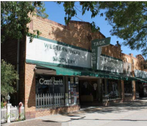
The Christesen's building was constructed at 629-633 Main Street in 1926.
