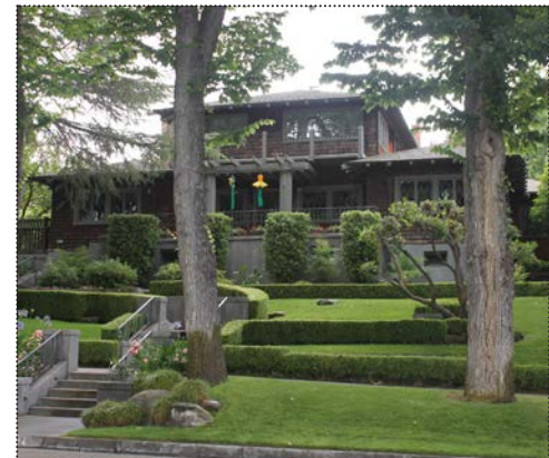
Craftsman-style residence at 4672 Second Street (ARG, June 2012).
