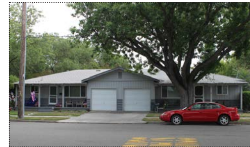
Multifamily dwelling unit at 104 Abbie Street (ARG, June 2012).
