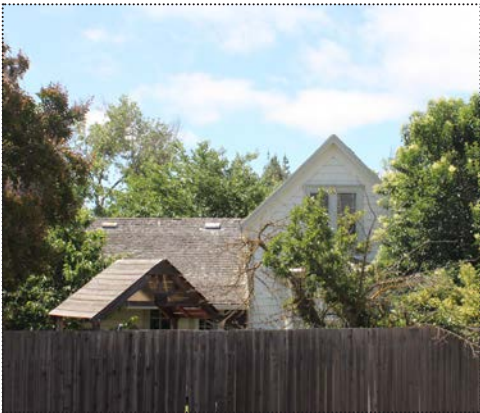
3988 First Street (ARG, June 2012).
