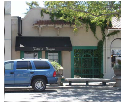
The Graham Mortuary at 706 Main Street was built in 1910 (ARG, June 2012).
