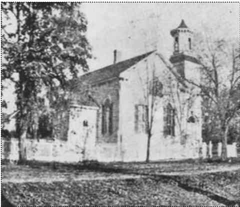
The First Presbyterian Church was built in 1876. The foundation was made of Pleasanton Company bricks (from Pleasanton . Images of America, 51).
