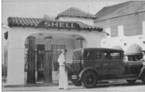
The J.J. Amaral Service Station and Garage were built in 1931 (from Pleasanton. Images of America , 123).
