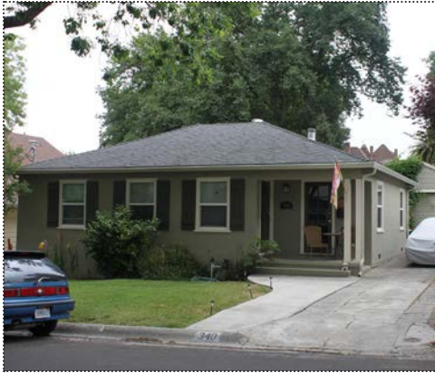
An FHA Minimum House at 340 East Angela Street (ARG, June 2012).
