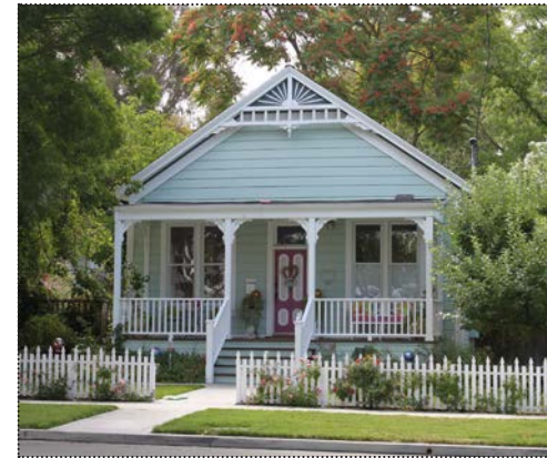
End gable residence at 4362 Second Street (ARG, June 2012).
