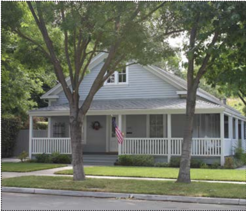
End gable residence at 4376 Second Street (ARG, June 2012).
