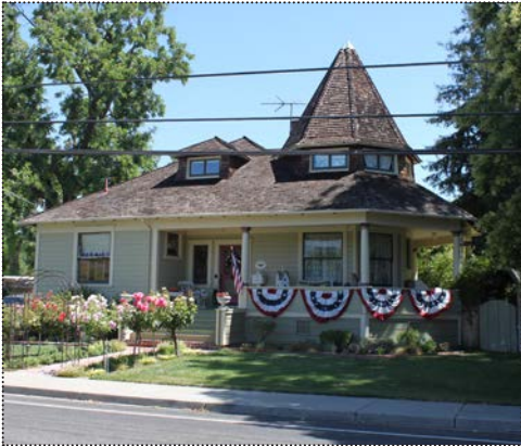
Residence at 733 Division Street was built in 1895 (ARG, June 2012).
