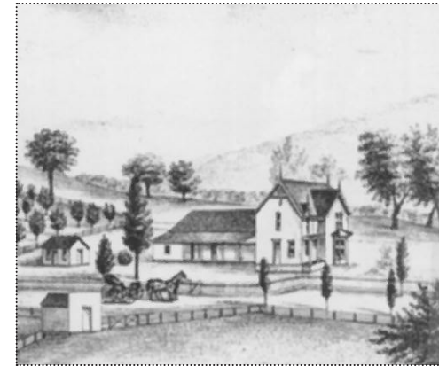
1878 sketch from Thompson and West's Historical Atlas showing the residence of Joshua and Angela Neal. A portion of this house remains at 431 Neal Street ((from Pleasanton . Images of America, 23)
