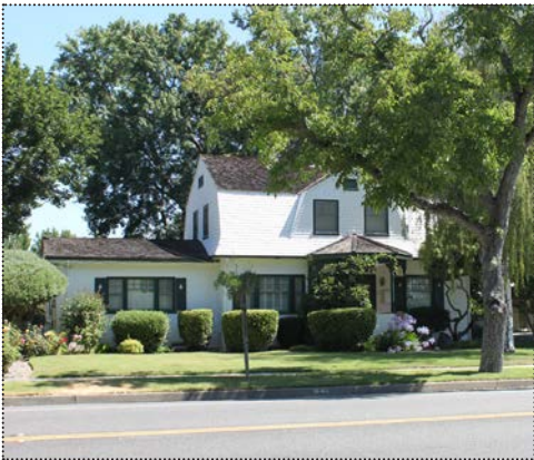
Bay Tradition residence at 621 St. Mary Street (ARG, June 2012).
