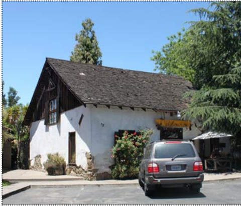
The John Kottinger Barn at 200 Ray Street was built in 1852 (ARG, June 2012).
