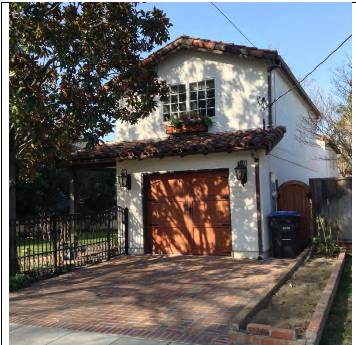
Garage addition, looking W
