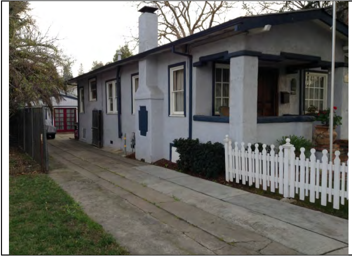
Looking SE from First Street
