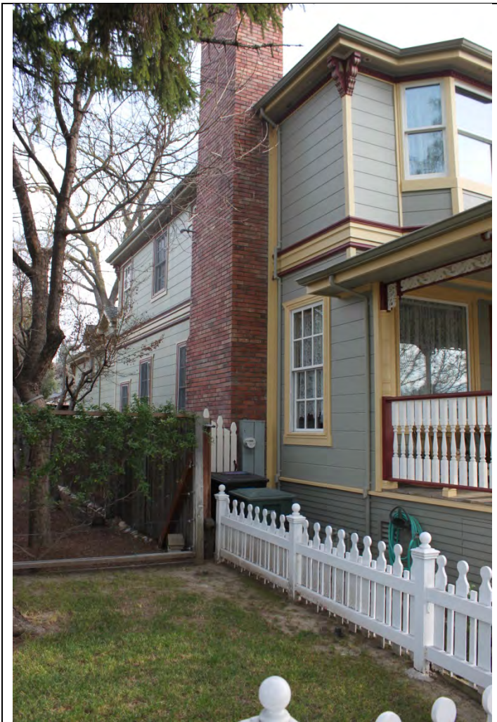
Looking SE from First Street
