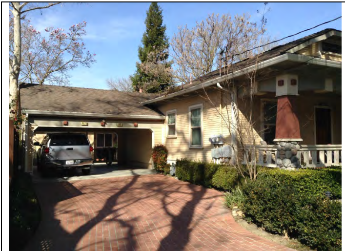
South elevation and porte-cochere Looking W from Second St.
