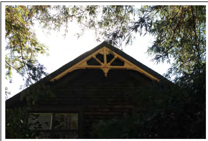
Detail, stick work on gable, north elevation
