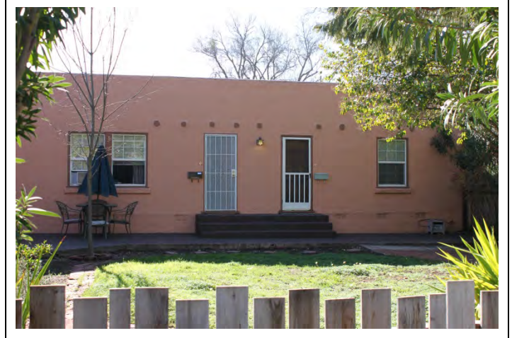
Detail, courtyard, looking S
