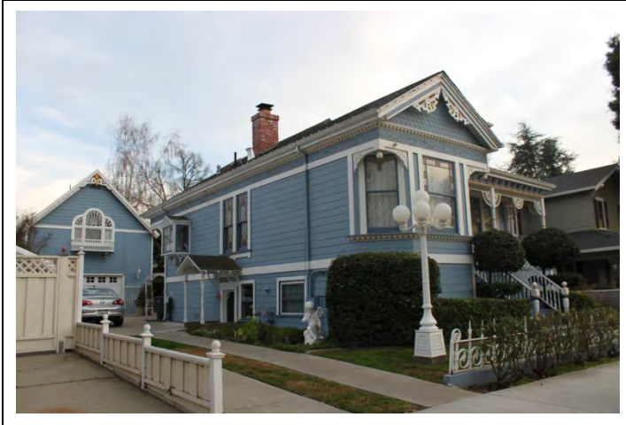
Looking SE from First Street
