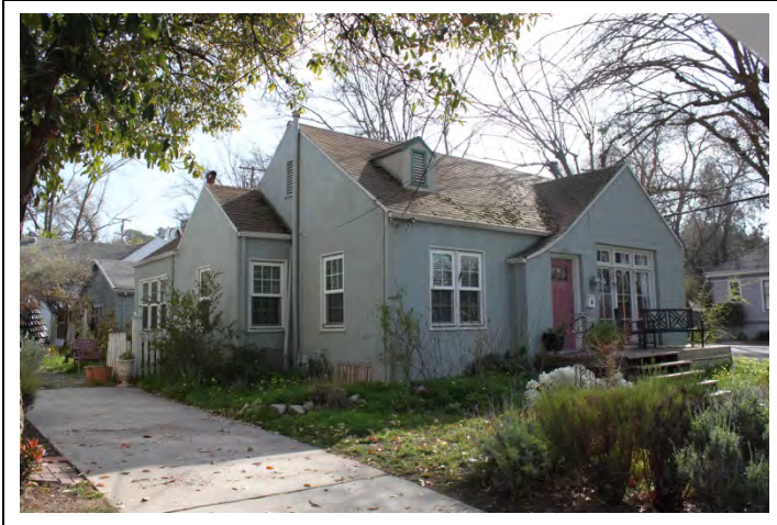
Looking SE from Second St.
