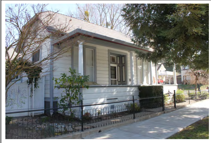
Original main elevation fronting on E. Angela St. Looking NE from E. Angela St.
