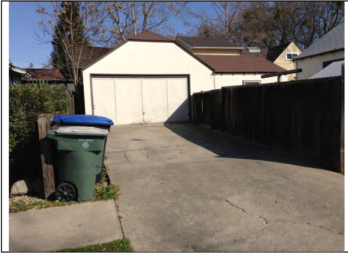
Garage, oriented to Abbie St.
