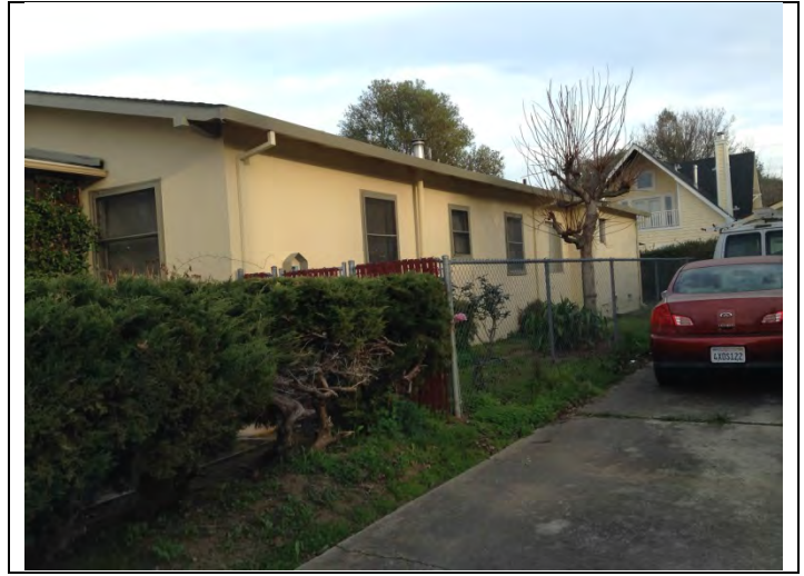
South elevation, showing rear addition Looking NE from First Street
