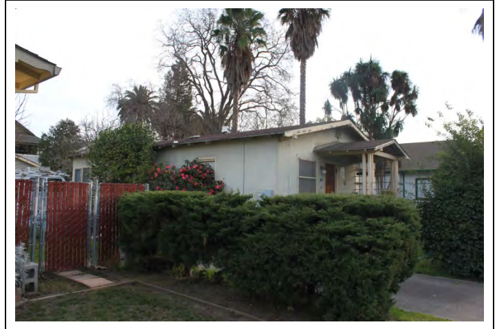
Looking SE from First Street
