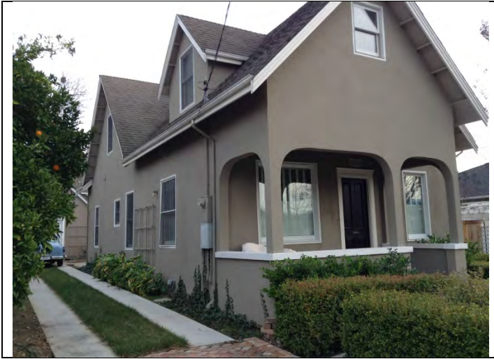
Looking SE from Second St.
