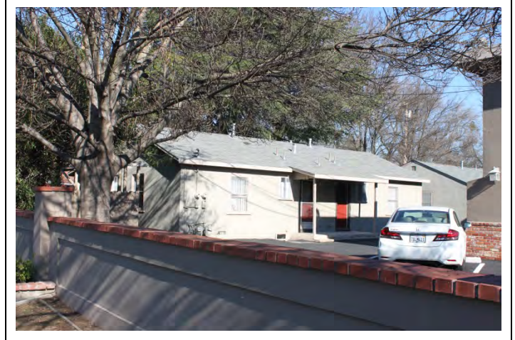
Rear (south) elevation, 470 Division Street Looking NE from Anderson St.
