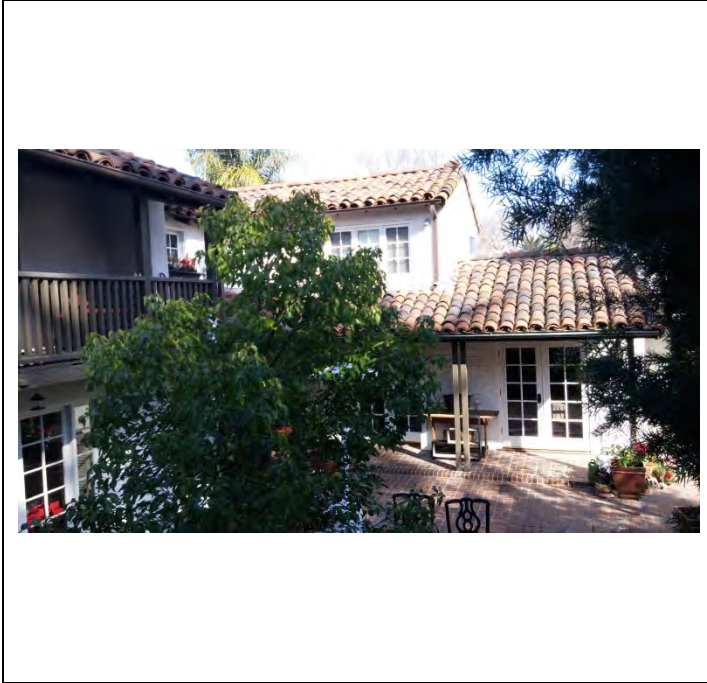
Looking N at 1997 addition
