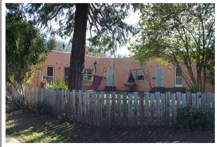
Looking SE from corner of First and E. Angela Sts.
