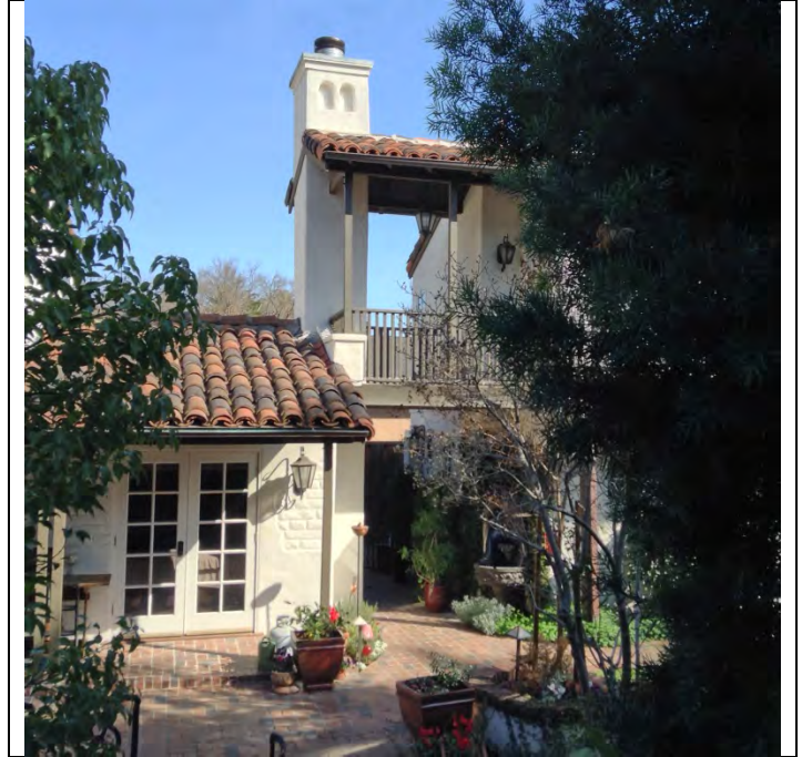
Looking N at 1997 addition
