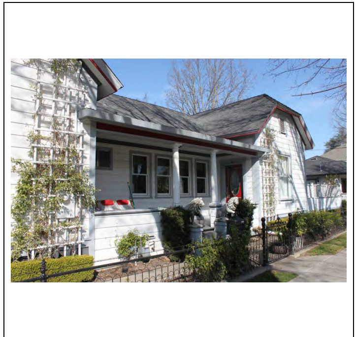
East elevation on Second St. Looking NW from Second St.
