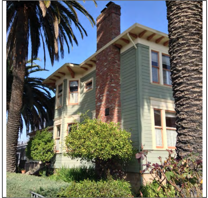
Looking NW from corner of Second St. and Arendt Way
