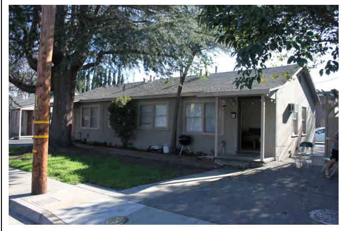
470 Division Street Looking SE from Division Street
