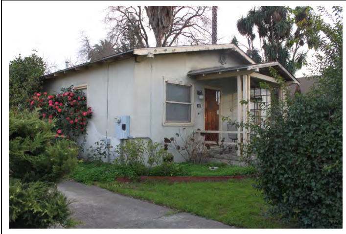
Looking SE from First Street
