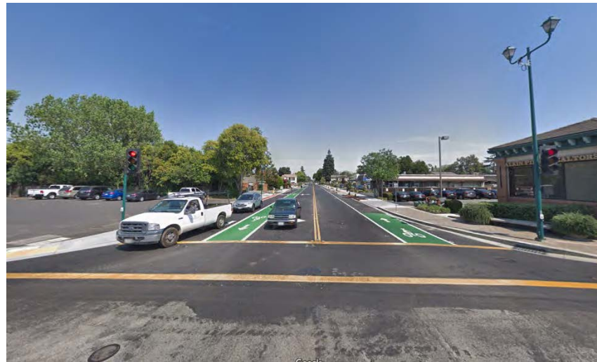
Stanley Boulevard east of Main Street
