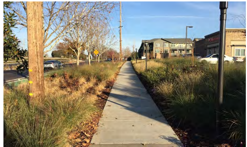
Existing six-foot sidewalk east of intersection needs to be widened to eight foot minimum, but preferably ten-foot/Class I
