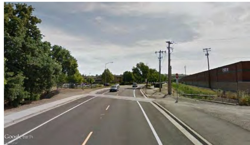
Crossing at Valley Avenue
