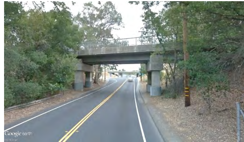
Overcrossing at Pleasanton-Sunol Road
