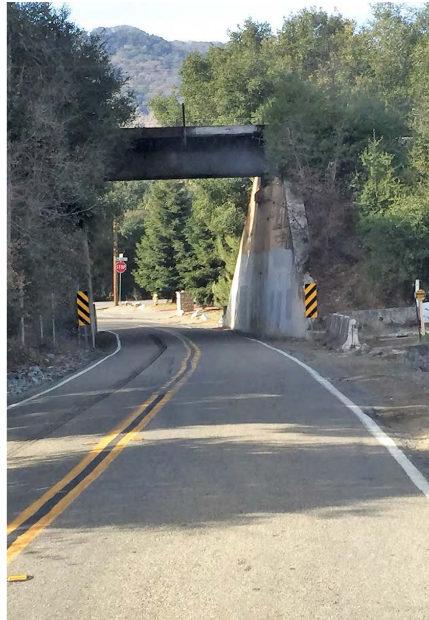
Narrow opening at trestle
