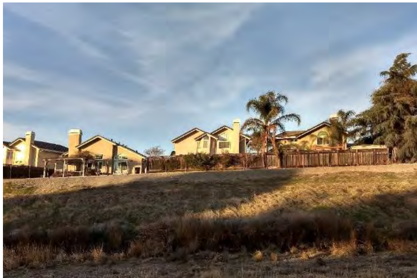
View of typical segment behind residences
