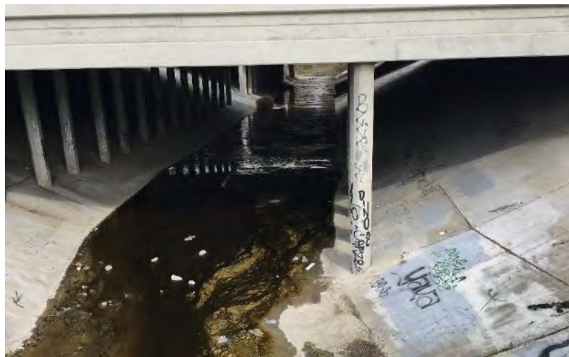
View north under I-580 at Tassajara Creek
