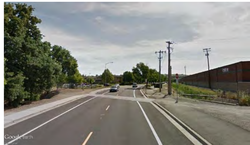
Crossing at Valley Avenue
