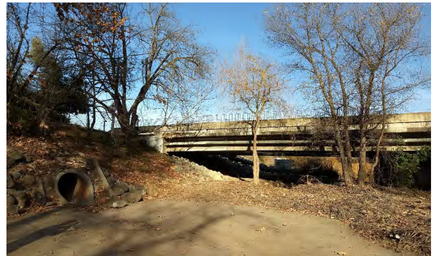
Low undercrossing at Bernal from the west
