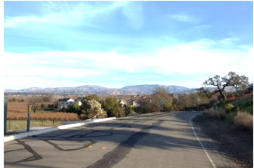
Section closed to vehicles southeast of Vineyard Terrace
