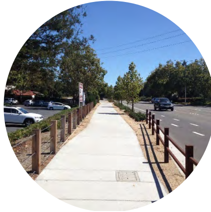
Class I Multi-Use Trail Along Roadway
