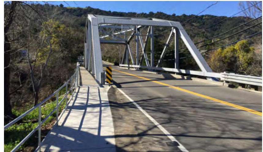
View from east side of bridge over arroyo at Bernal
