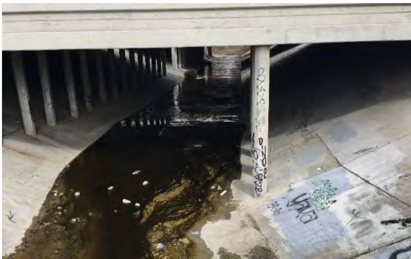
View north under I-580 at Tassajara Creek
