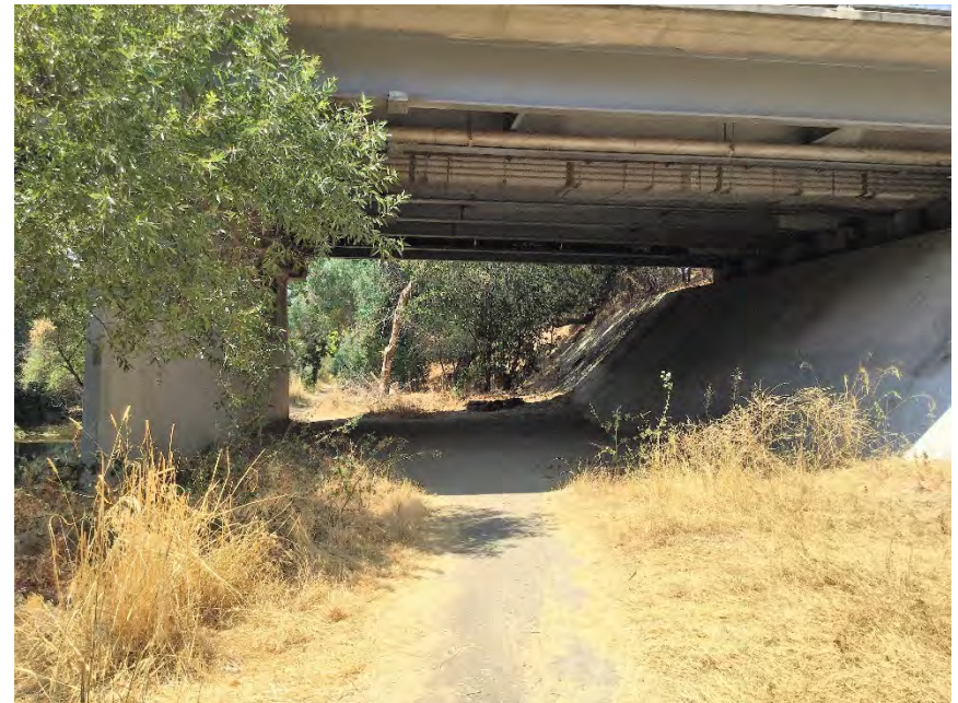
Undercrossing and street connection at Valley Avenue
