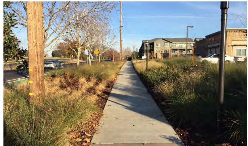
Existing six-foot sidewalk east of intersection needs to be widened to eight foot minimum, but preferably ten-foot/Class I
