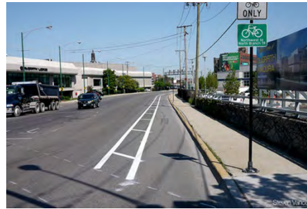
Buffered bicycle lane with wayfinding signage
