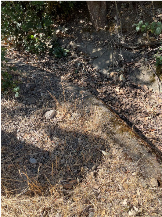
ID OTF-9: Leaves accumulated in concrete drainage ditch.
