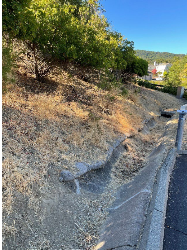
ID LC-10: Slow drainage of catch basin during rain events.
