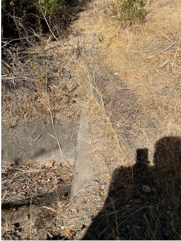
ID OTF-1: Erosion rill on slope and access road, jute fabric placed on slope for erosion control.
