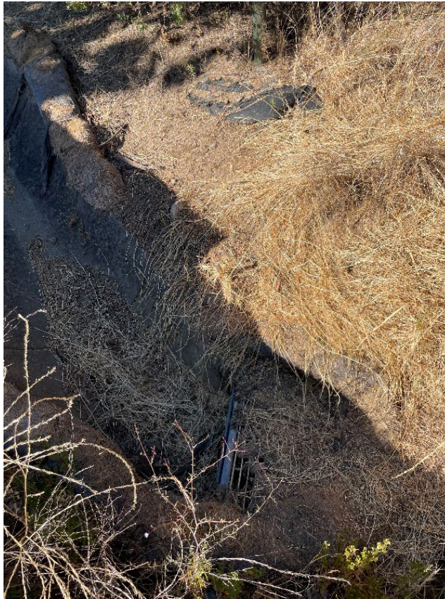
ID LR-16: Leaves and branches accumulated in earthen ditch.
