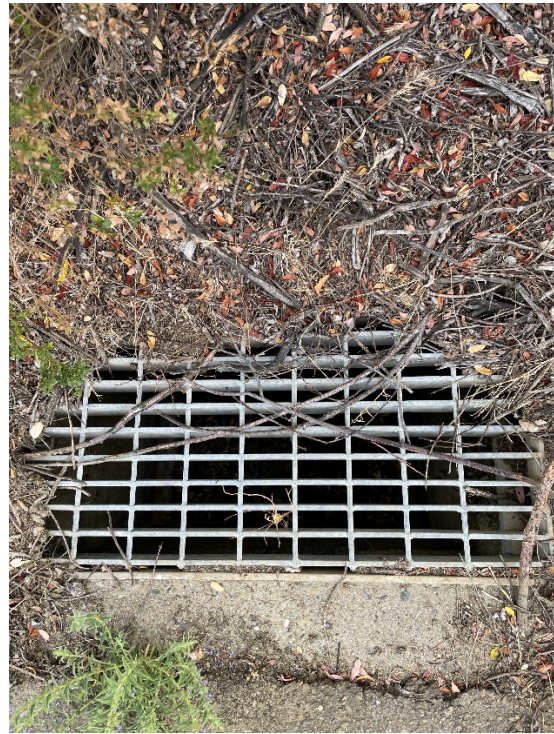
ID MR-30: Debris accumulated at drain inlet on north side of road.
