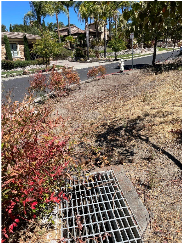
ID LC-10: Slow drainage of catch basin during rain events.
