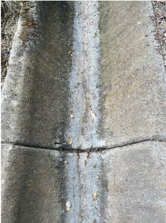
ID MR-18: Cracking and offset in concrete-lined drainage ditch. Soil accumulated in concrete-lined drainage ditch.
