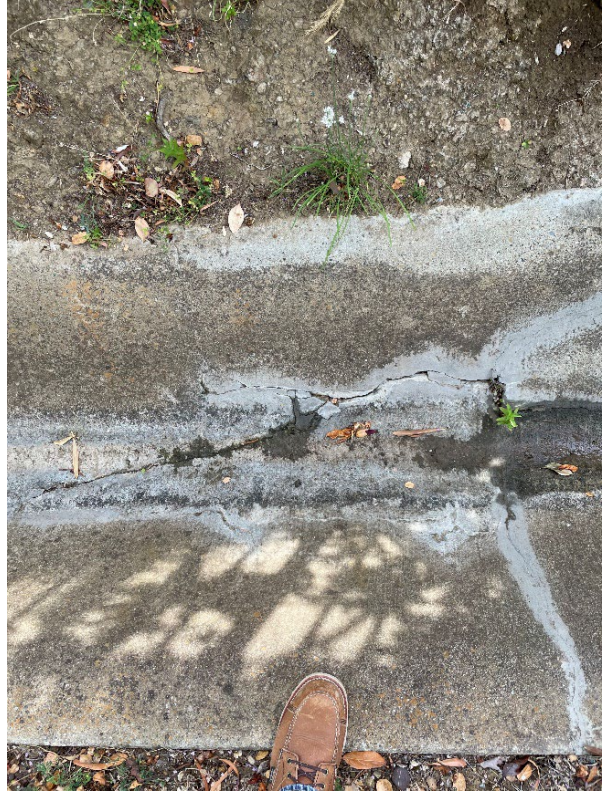
ID MR-6: Cracking in concrete-lined drainage ditch.
