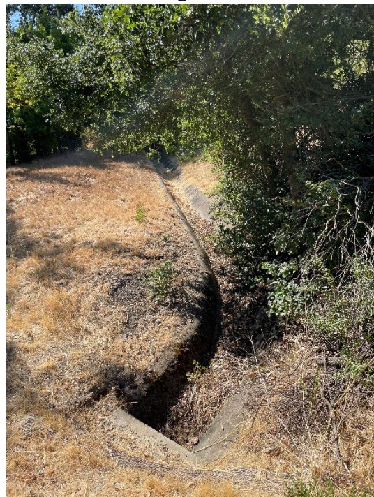
ID OTF-9: Leaves accumulated in concrete drainage ditch.
