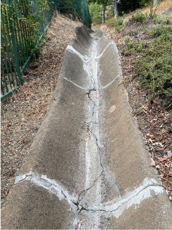
ID MR-6: Cracking in concrete-lined drainage ditch.
