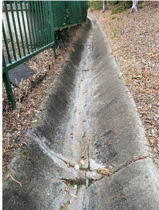
ID MR-18: Cracking and offset in concrete-lined drainage ditch. Soil accumulated in concrete-lined drainage ditch.
