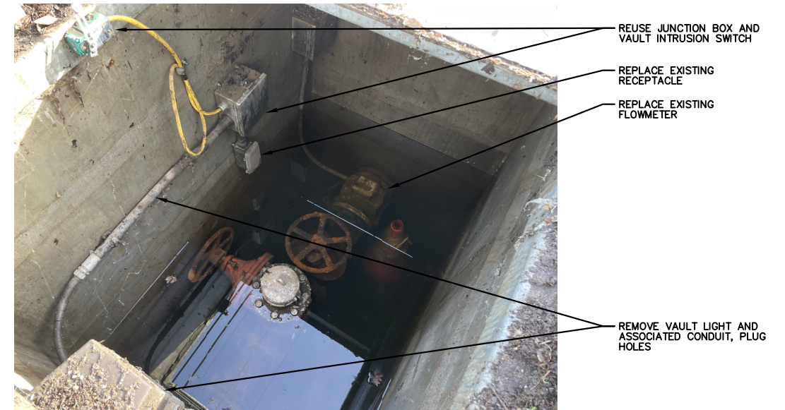
FLOWMETER VAULT PHOTO ①
