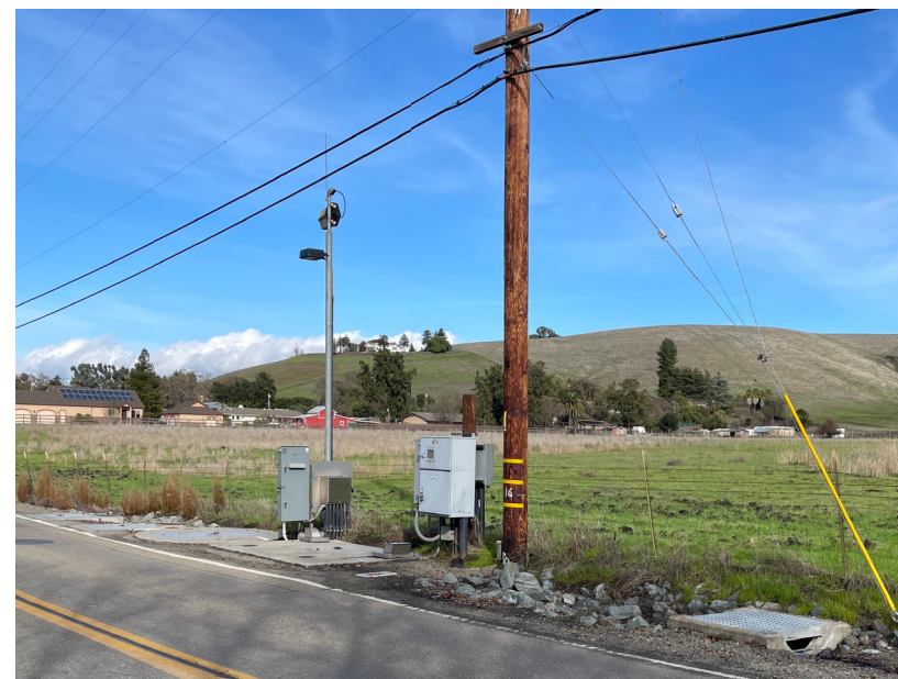
EXISTING LIFT STATION PHOTO
