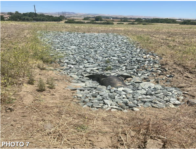
VIEW OF DRAIN ROCK AND CULVERT NEAR THE WESTERN PERIMETER OF SITE
