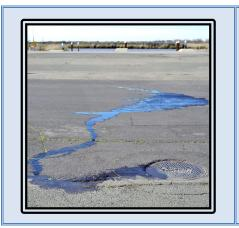
Identify the point of the spill where the wastewater entered the waterway and take a photograph of this location with a reference point in the picture.
