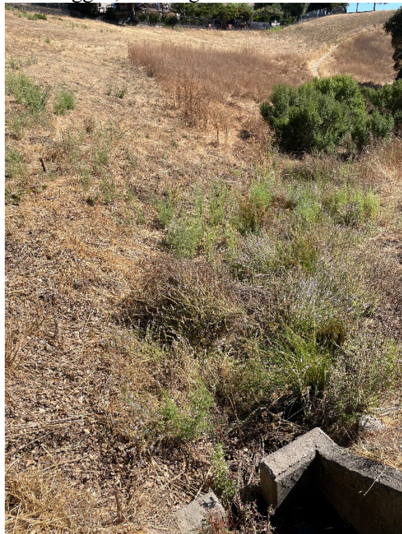
ID LC-23: Drainage inlet in open space is clogged, standing water in DI.
