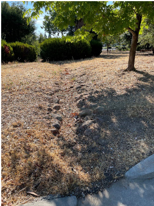
ID LR-7: Existing grade does not drain to gutter pan.
