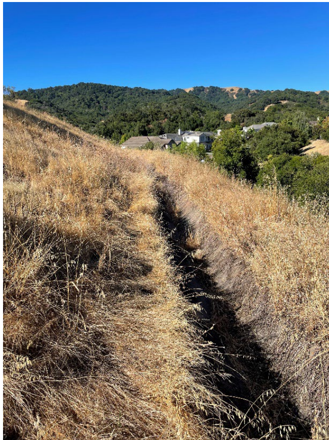
ID LC-18: Overgrown vegetation on sides of V-ditch. Leaves and grass accumulated in concrete-lined drainage ditch.
