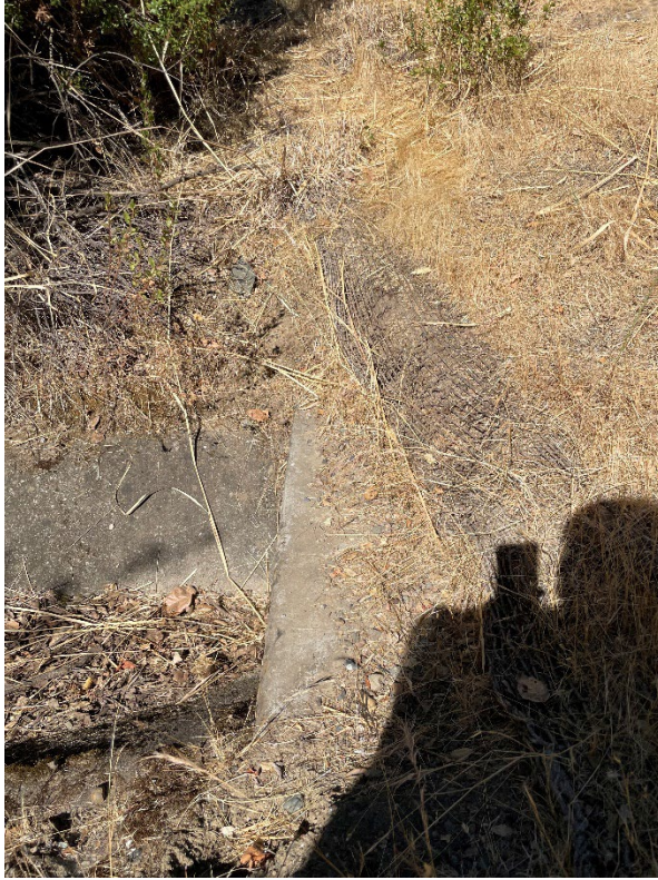
ID OTF-2: Storm drain clogged.
