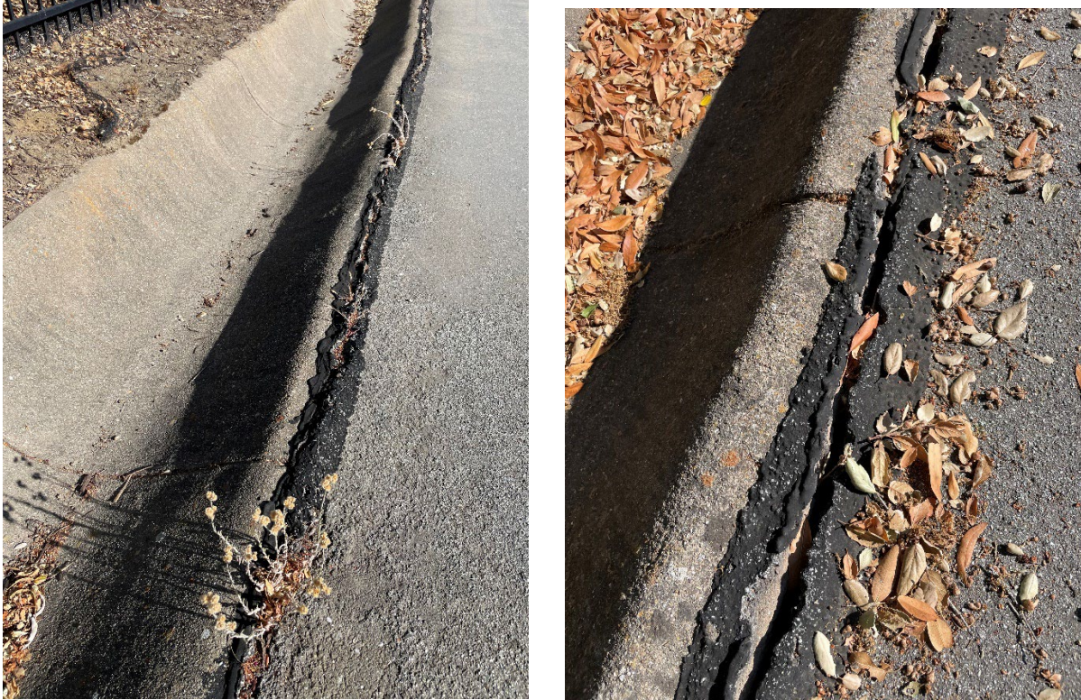
ID LC-18: Overgrown vegetation on sides of V-ditch. Leaves and grass accumulated in concrete-lined drainage ditch.
