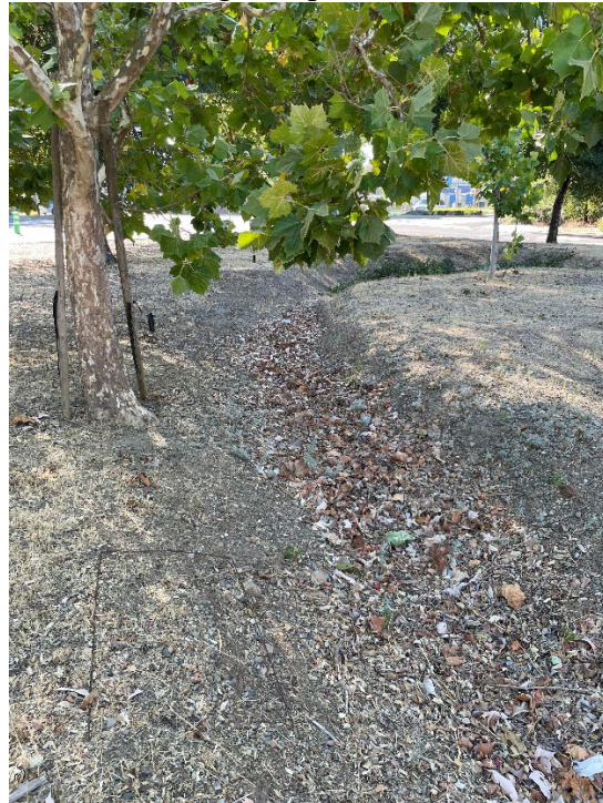
ID LR-7: Existing grade does not drain to gutter pan.
