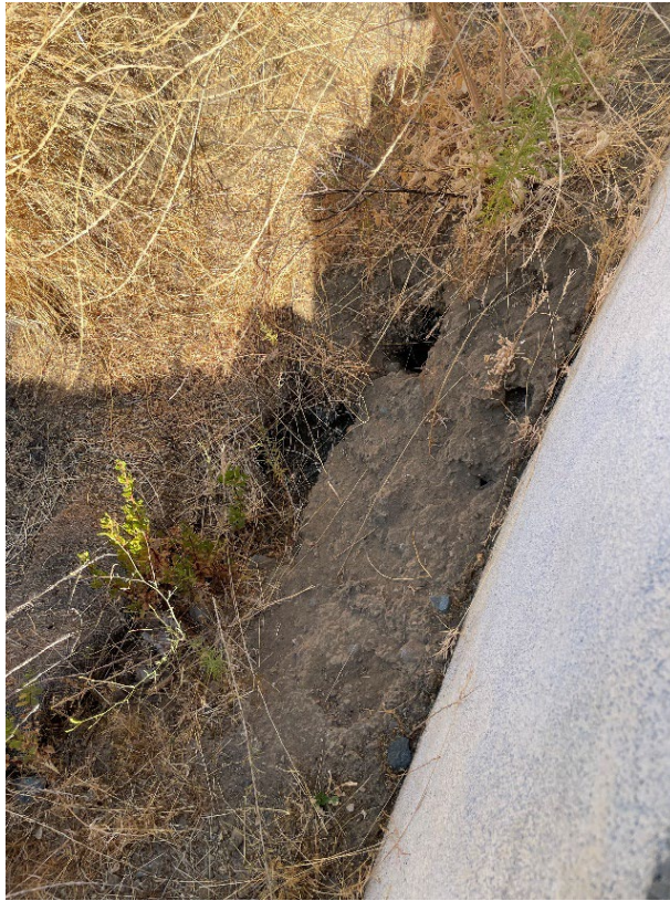
ID LR-7: Existing grade does not drain to gutter pan.
