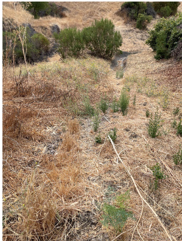
ID MR-9: Ditch segment buried with soil and vegetation.
