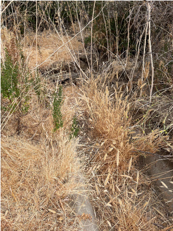
ID MR-9: Ditch segment buried with soil and vegetation.
