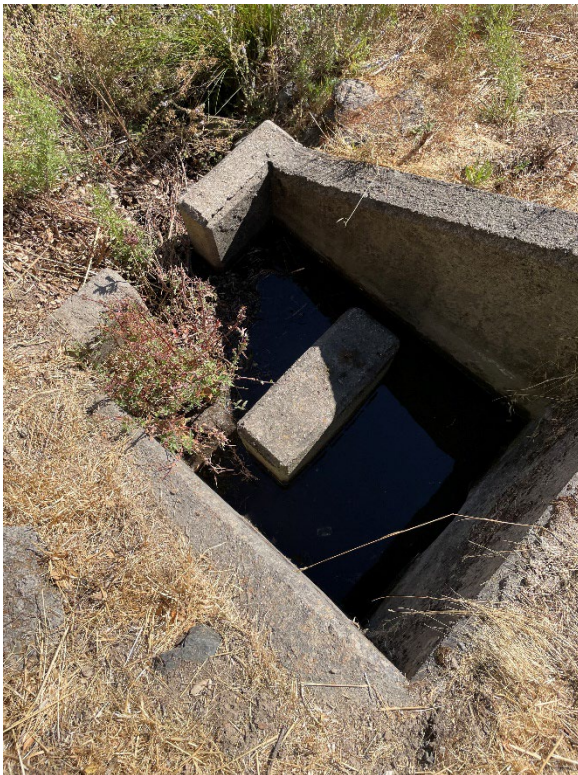
ID LC-23: Drainage inlet in open space is clogged, standing water in DI.
