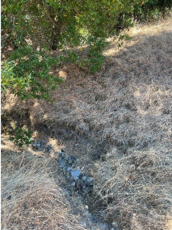
ID LC-36: Erosion at outfall of SD-11, area overgrown with dense grasses and weeds.
