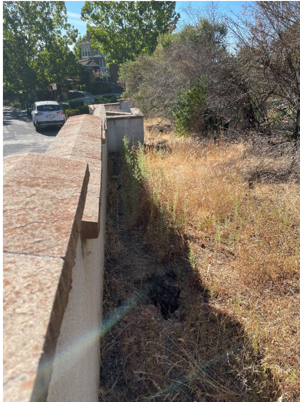
ID LR-1: Animal burrowing created a void behind wall.
