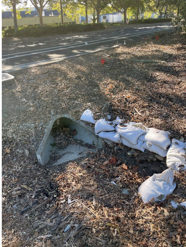
ID LR-19: Sand bags installed around field inlet
