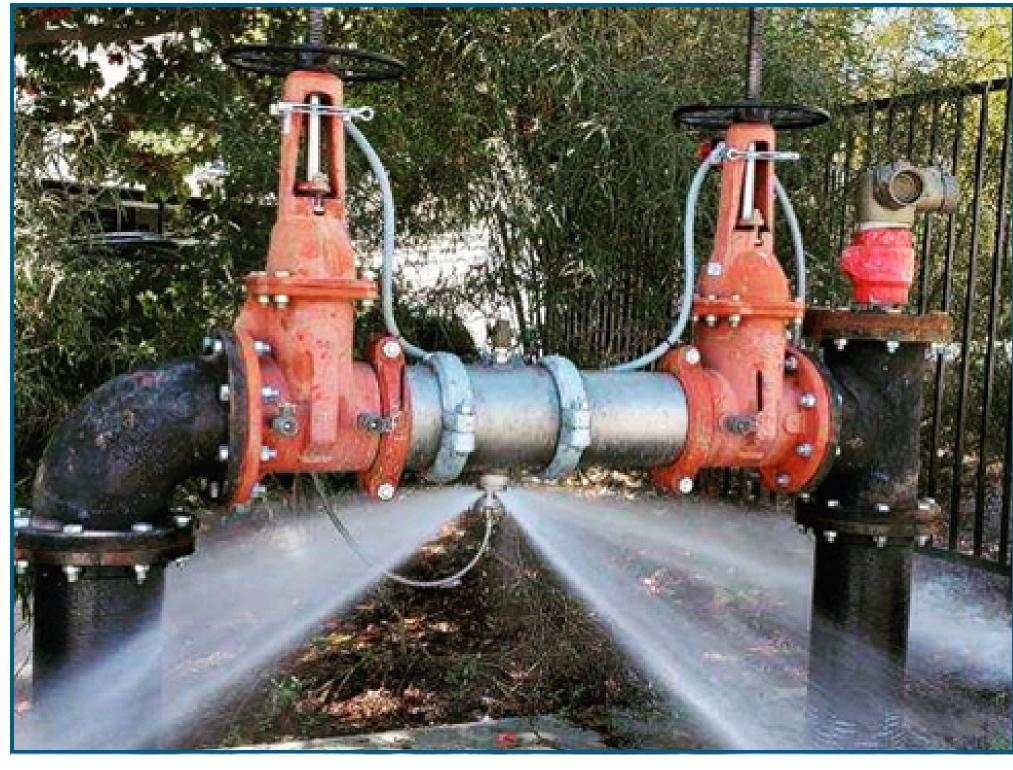
Backflow Inspection & Maintenance: Devices are regularly inspected and repaired to prevent backflows into the water system.
