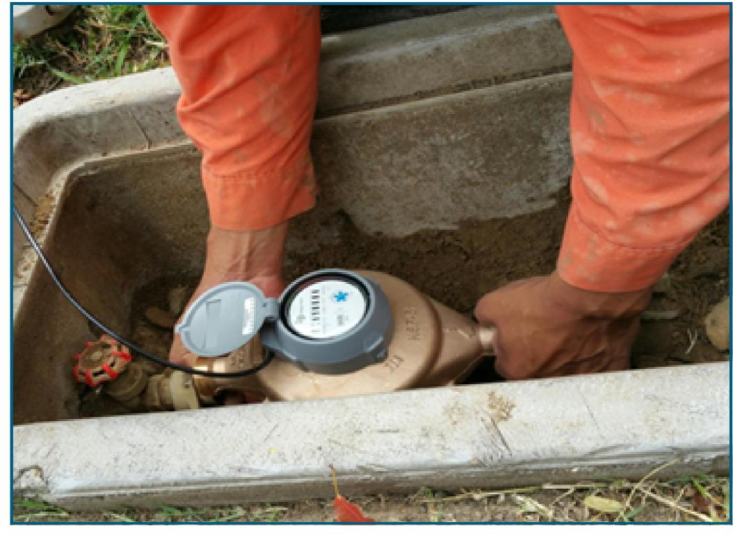
Water Meter Repair: The City maintains approximately 22,000 water meters. Currently, the City is replacing an average of 250 meters each month.
