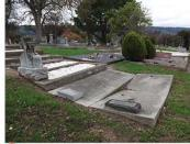
18 SINKING GRAVE COVERS Decaying caskets are causing grave covers to crack and sink. In some cases this creates tripping hazards and should be repaired or re-
